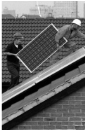
Installing solar panels
